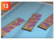
Try and limit the amount of walking on the boards, and where possible lay boards to prevent indentations on the boards.
