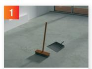
Remove all contaminants, dirt, grease etc. from the substrate and make dust free.
