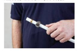
**Step 4:** Insert the brass body of the connector into the pipe.
